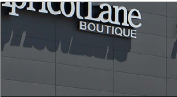
THIN BRICK PANEL SIDING - BRK-1 BRAND: NICHHA COLOR: STEELE FINISH: TUFFBLOCK
