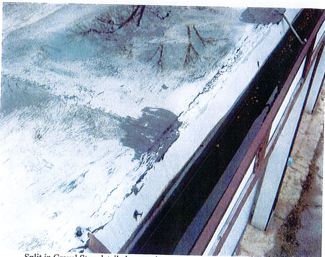
Split in Gravel Stop detail along perimeter edge allowing water into system
