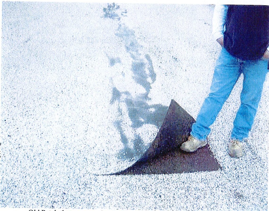
Old Patch that you can simply lift up by hand allowing moisture under
