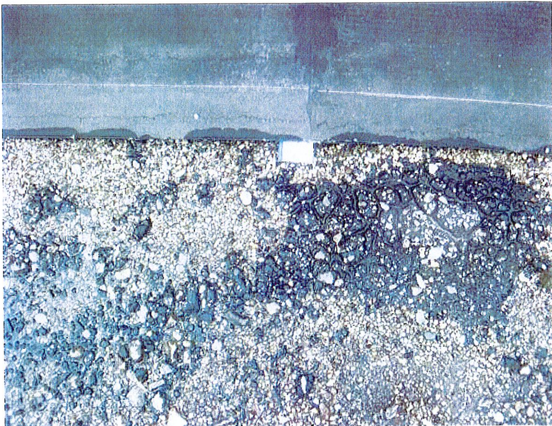
Entire length of Modified Bitumen flashing detail not adhered at base
