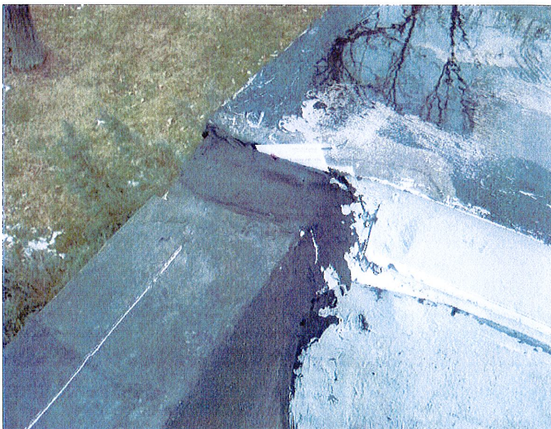
Opening in Gravel Stop detail where two roofs meet
