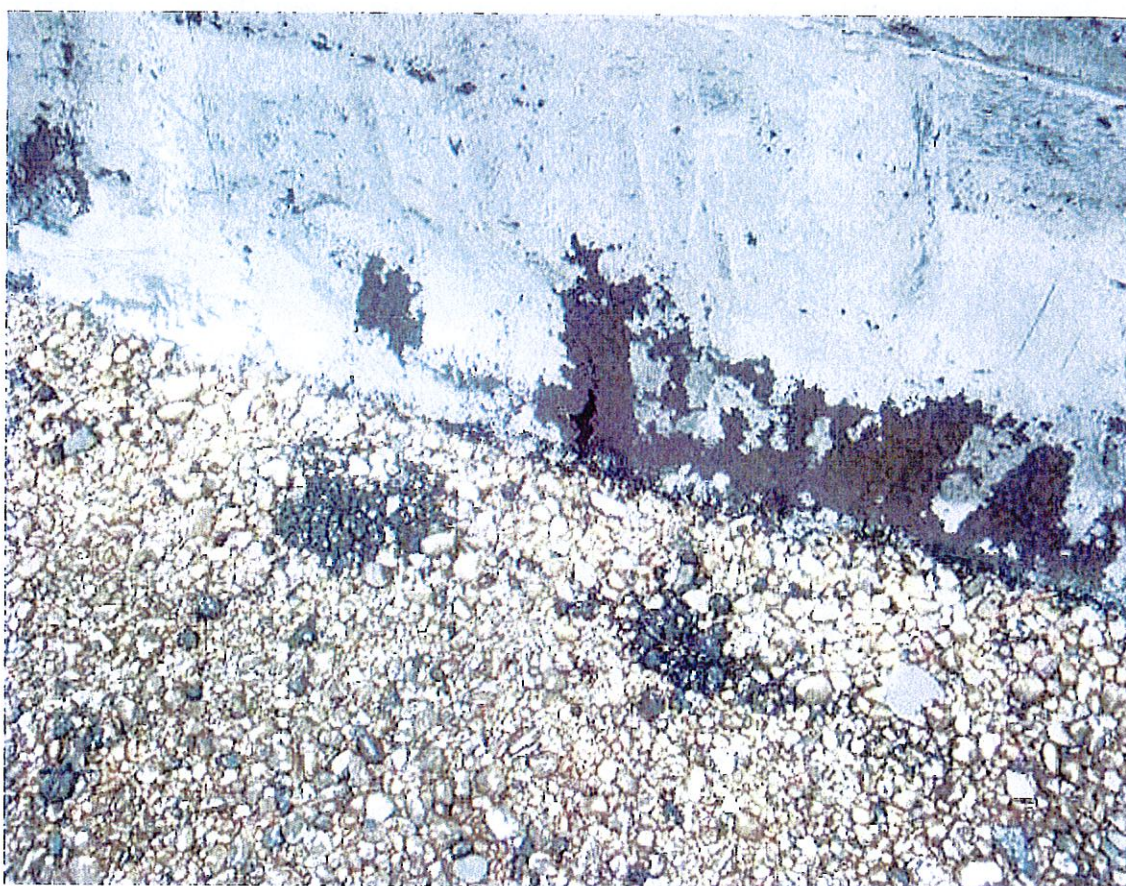
Another section of broken down flashing detail
