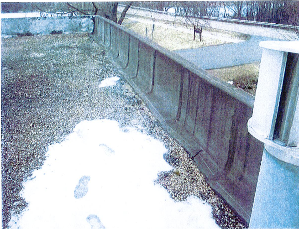
Overview of Parapet Wall Flashing detail on front of building
