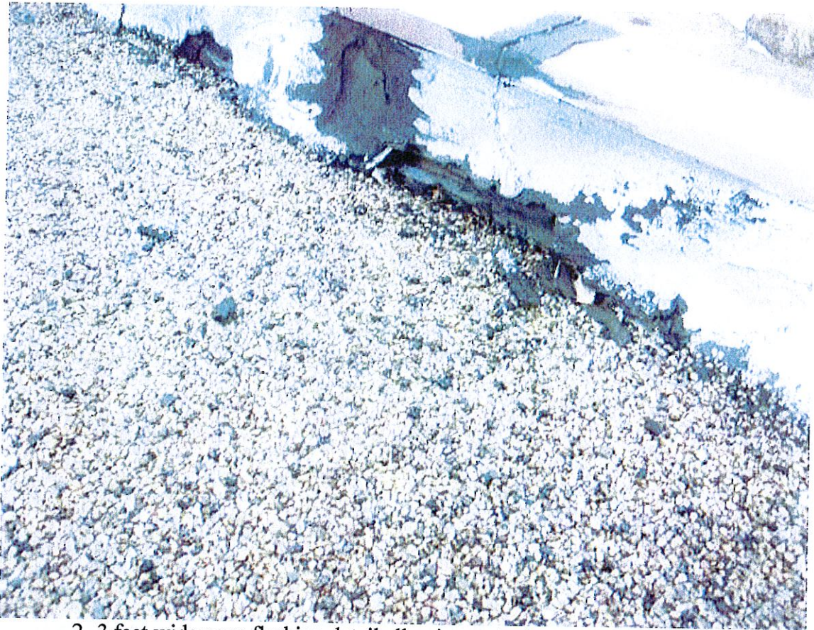
2 -3 feet wide open flashing detail allowing water into system or building
