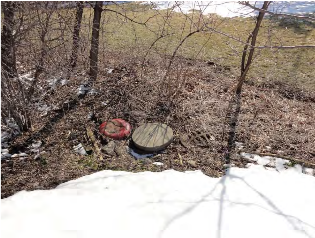
Blocked manhole/catch basin along the east side of the tracks 300 feet north of Main Street in Study Area B
